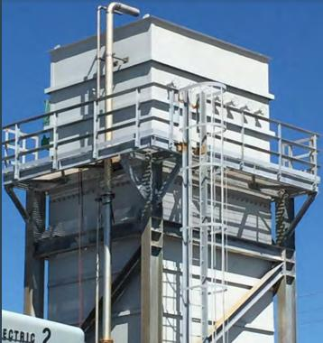
Moran Iron Works was awarded the contract to fabricate and deliver a new Frame 5 silencer. The work also included demo of the old silencer unit and installation of the newly fabricated one. This unit was shipped via oversized load to Stock Key / Key West in one piece with lifting lugs installed for both rolling and lifting. Plenum repairs were also required due to years of degradation in the salt water environment.
